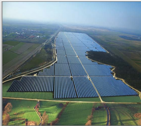
Karadzhalovo, Bulgaria – 60 MW
